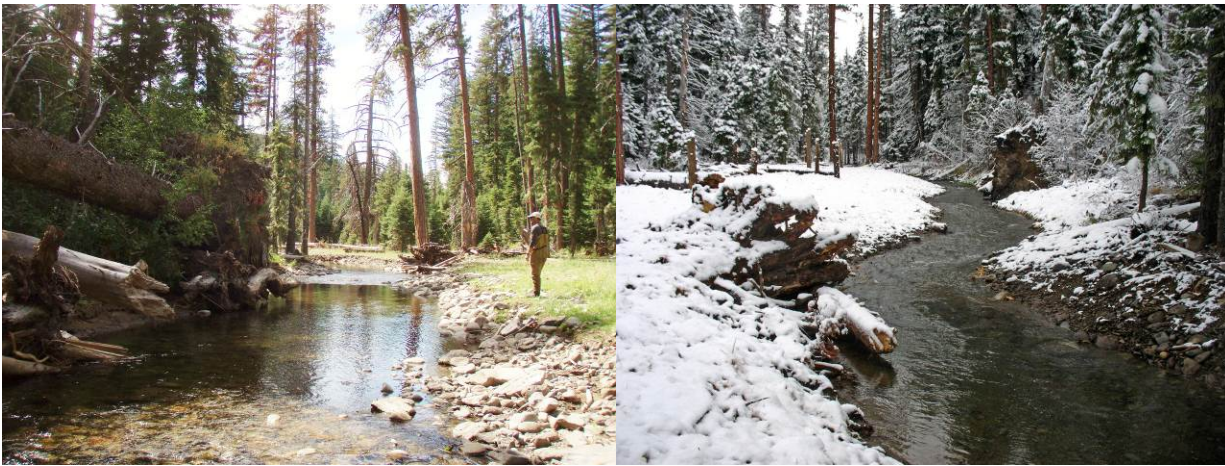
Figure 4. Constructed portion of side channel (approx. 2000').
